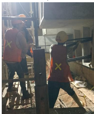
Gambar 10. Instal Kabel Strand
