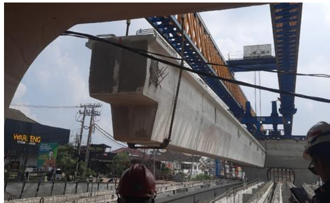
Gambar 17. Loading Test Girder
