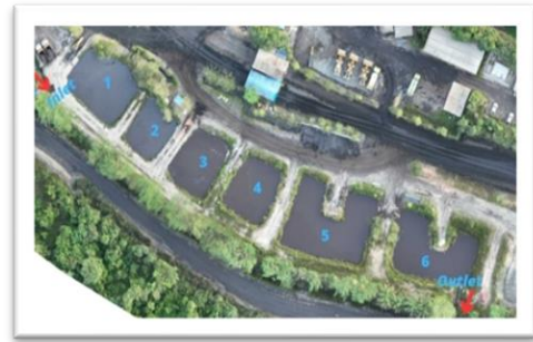
Gambar 1 SP Crusher II
